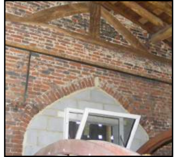
Refurbished bell tower with sound proofing
